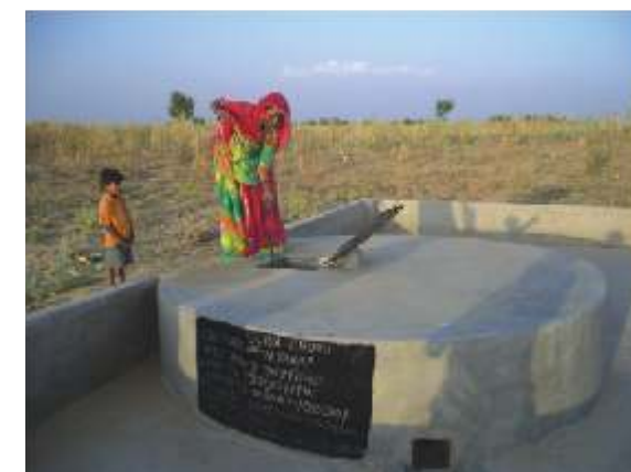
Nathu Kanwar's surface water harvesting tankaa at Sajansar, Bikaner
